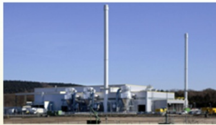
Mechanical & Biological Treatment Plant
