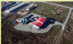
Kozani Waste Transfer Station
