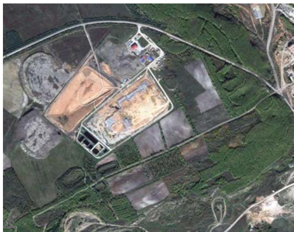
Imprinting plot, ACE construction and landfill
